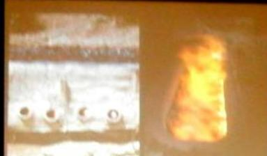
note intensity of fire inside front wall and flame over rim of front wall
